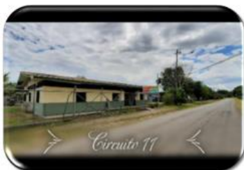
Control Interno Circuital
